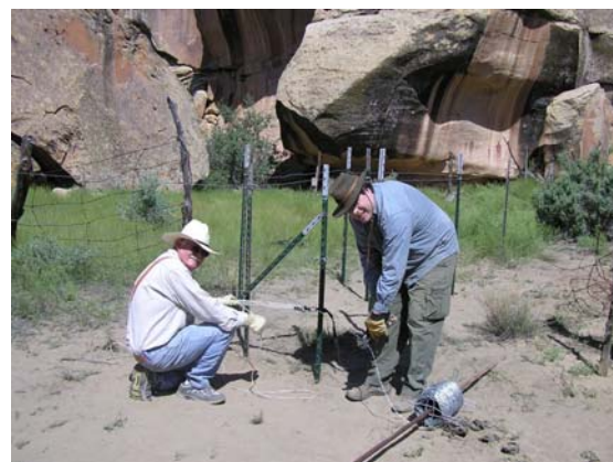
Quent and Troy tightening wire.
